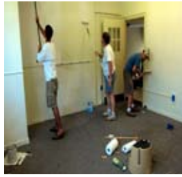
Painting one of the temple classrooms
